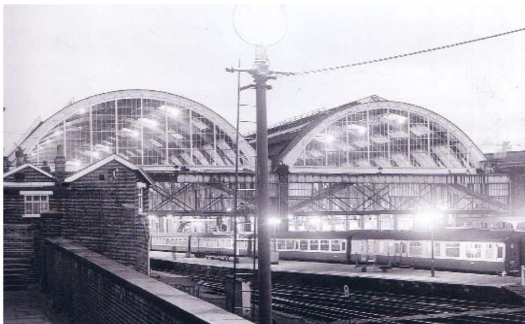
View of the south end of the Main Shed showing the framework for the original access bridge from the Eastern to the Western Range Buildings. The framework was removed by the 1970s.
